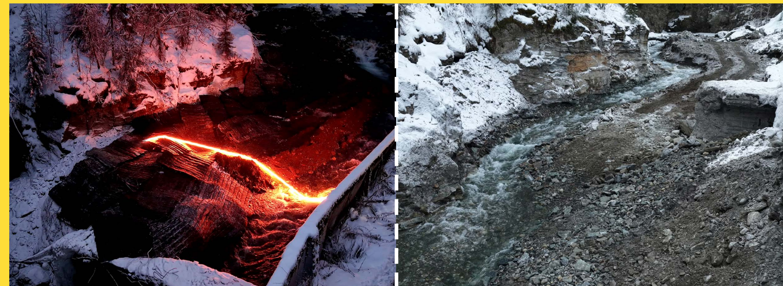
Figure 8. (left) Detonation of explosives during the removal of a dam on the Vinstra River, Norway, and (right) restored site after the dam removal © Kjetil Rolseth
