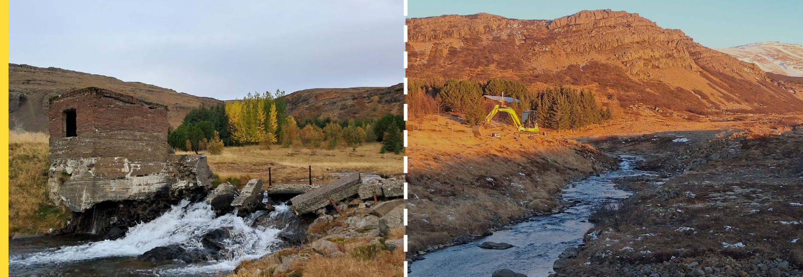
Figure 6. The Ytri-Hraundalur hydropower dam site at Melsá River in Iceland, (left) before and (right) after the removal works © (left) Jóhannes Guðbrandsson, and (right) Iðunn Hauksdóttir
