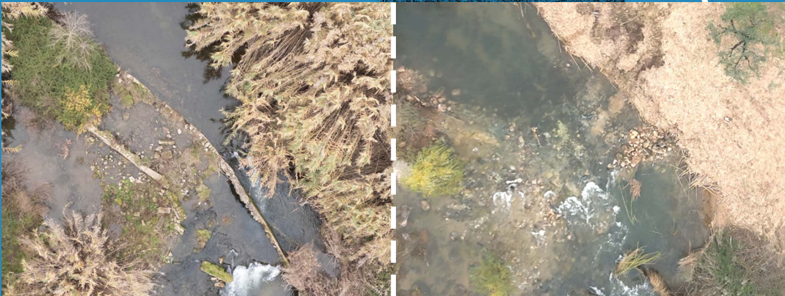
SOURINHO DAM – ALVIELA RIVER – PORTUGAL © GEOTA ( link )
