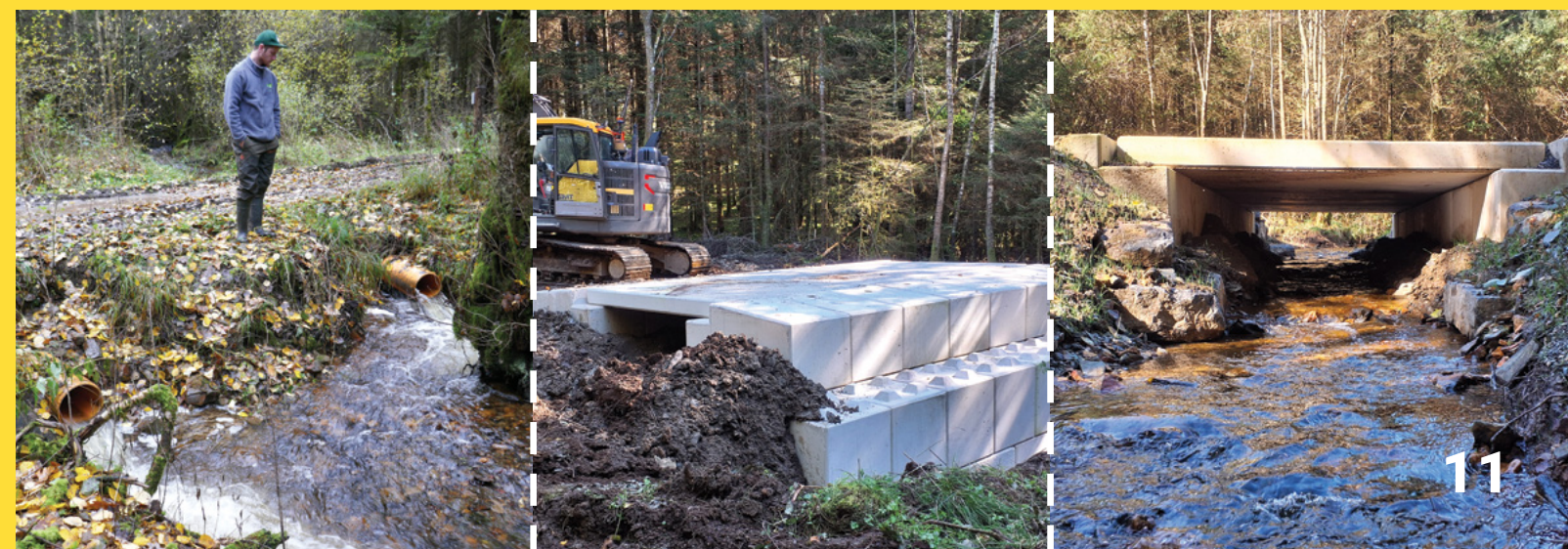
Figure 6. Pioneer culvert replacement technique by a bridge made of prefabricated blocks in Belgium © Parc naturel Haute-Sûre Forêt d'Anlier
