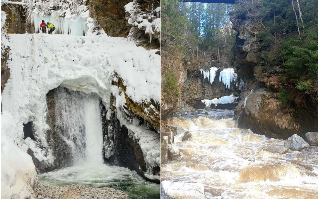
Dam on river Tromsa (Norway) before and after removal.
