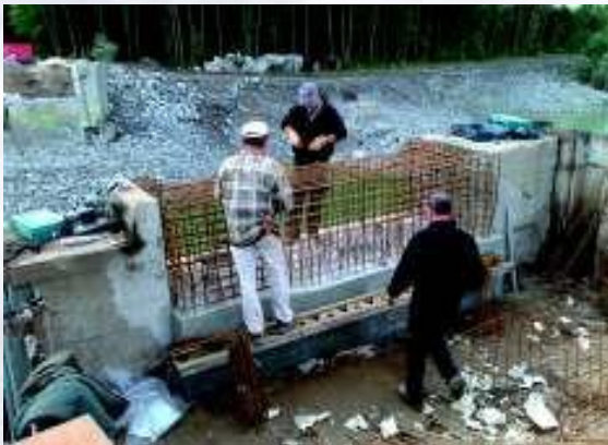
Renovation and adaptation of bridge abutments.
