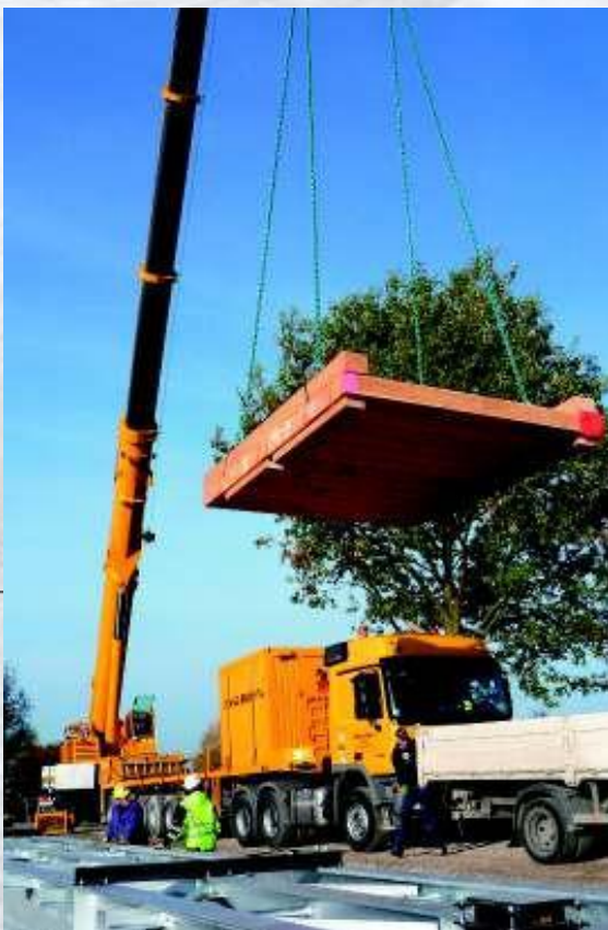
Fitting the new bridge superstructure.
