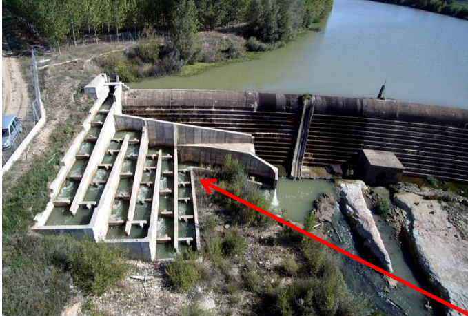
Pool-type fishway with notches and orifices
