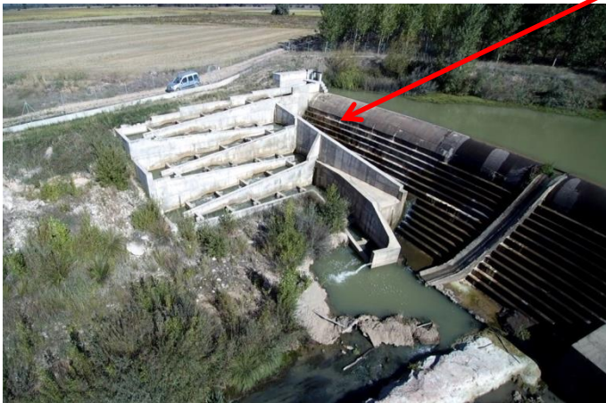
Pool-type fishway with notches and orifices
